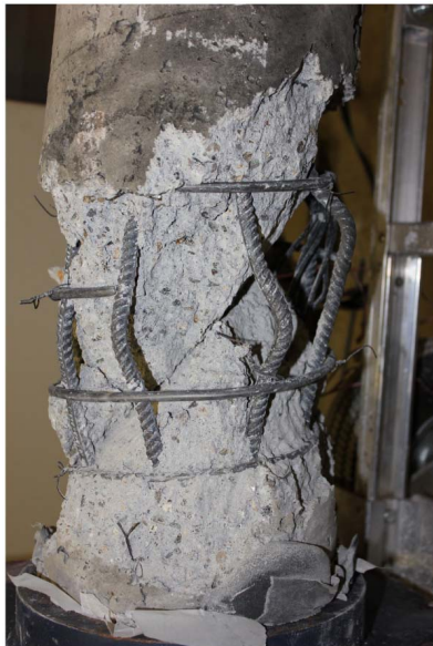
Fig. 13. Failure of the RC column under axial loading due to a shear crack initiated under blast loading (image by Arash E. Zaghi)
