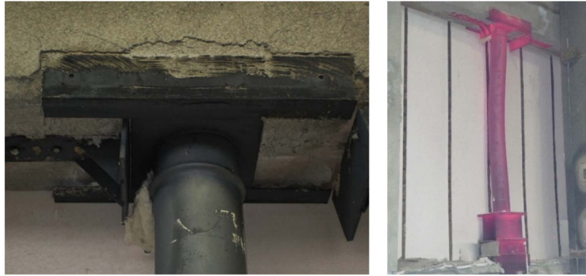
Fig. 11. Local and global buckling of specimen columns tested in fire (images by Michel Bruneau)
