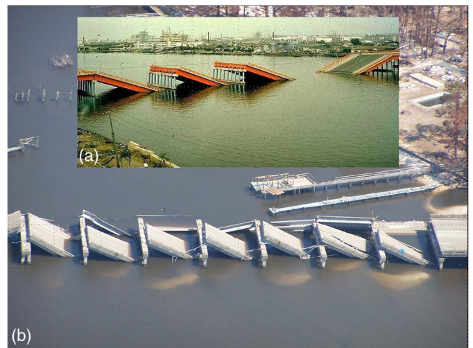
Fig. 1. Similarities in bridge span collapses observed: (a) after the 1964 Niigata earthquake (reproduced from Steinbrugge Collection, NISEE-PEER, University of California, Berkeley, with permission from NISEE-PEER); (b) following the 2005 Hurricane Katrina storm surge near New Orleans (across Lake Pontchartrain) (reprinted from O'Connor and McAnary 2008, photo used with permission, courtesy of MCEER)
